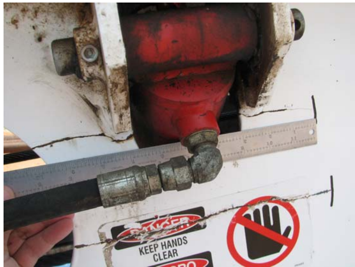
Figure 1- Example of cracks on the "Off Driller Side"
