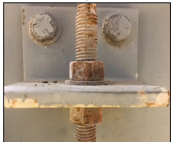
Figure 3: Correct Tensioning Spring Bracket and Fastener Orientation
