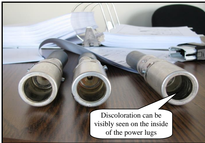
Figure 2: Discoloration on the inside of the power lugs
