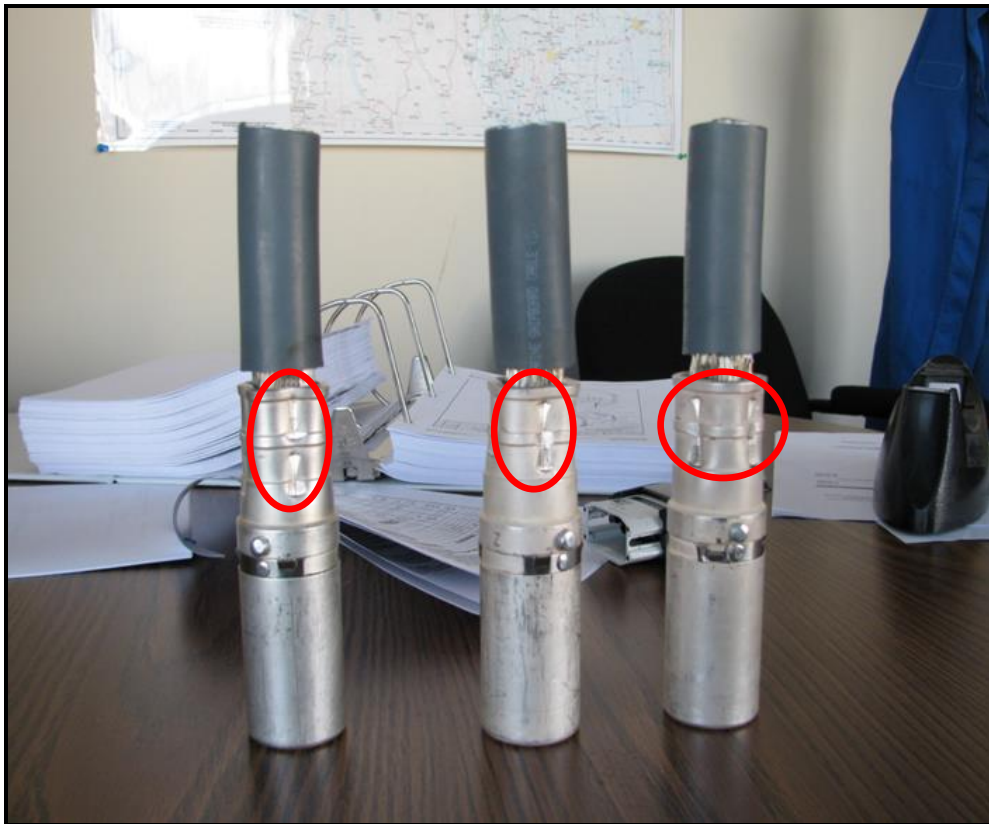
Figure 1: Cables improperly crimped at the lugs using a four-point crimp style
