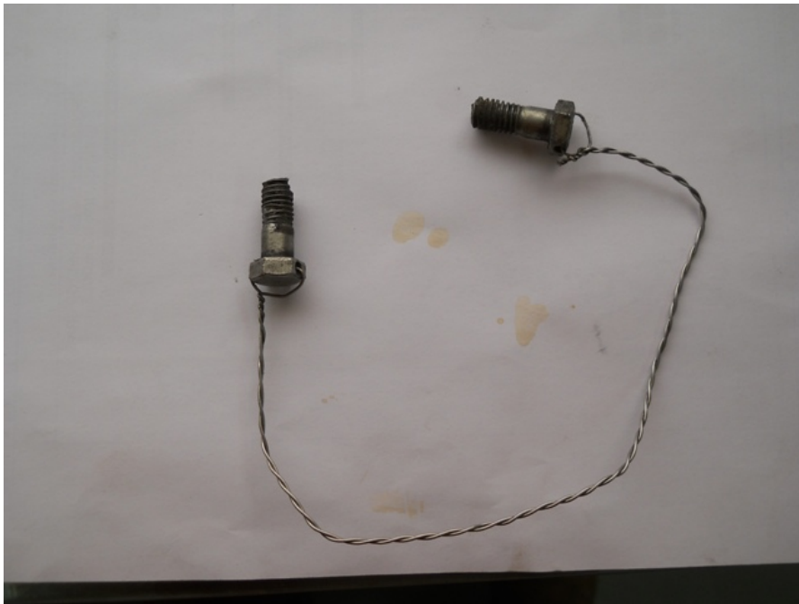
Figure 1 - Bolts that have come loose and fallen off an ESI 500 Ton Top Drive
