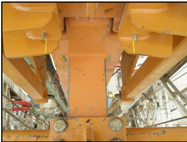
Figure 1: Upper T-bar secured with bolted clamp plate
