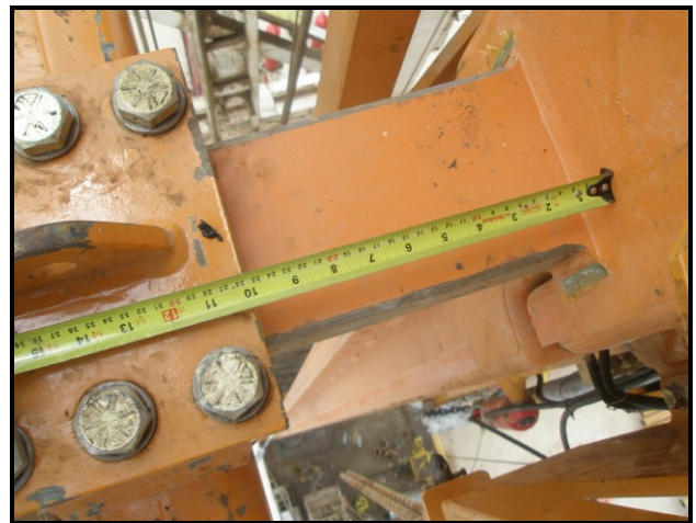
Figure 1: Upper T-bar secured with bolted clamp plate
